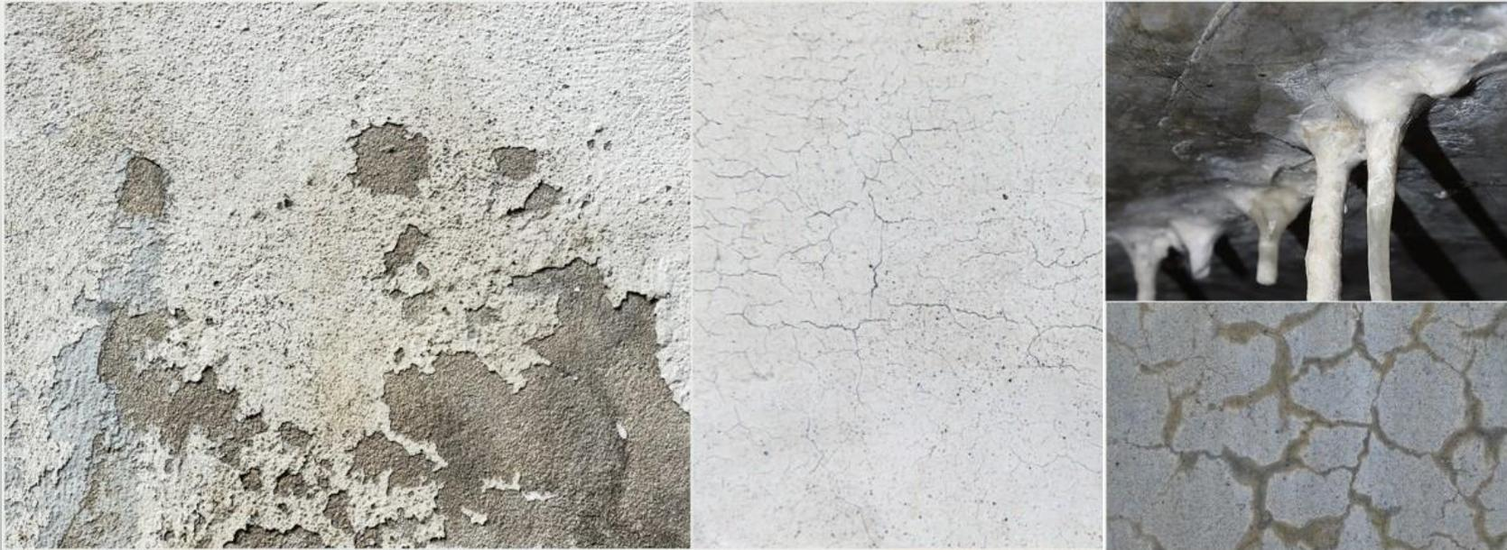
***“PERMEABILITY OF CONCRETE CAN BE A PRIMARY REASON FOR CONCRETE DETERIORATION DUE TO REINFORCING STEEL CORROSION AND OTHER DETERIORATION MECHANISMS.”***
